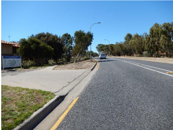
Photo 7-poor left hand sight line from Housing Trust driveway
