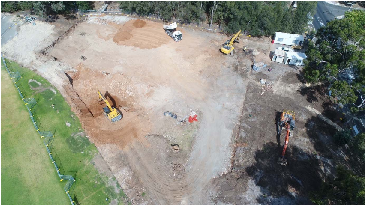
Figure 7, Aerial photo 2 March 2021, civil works commencing
