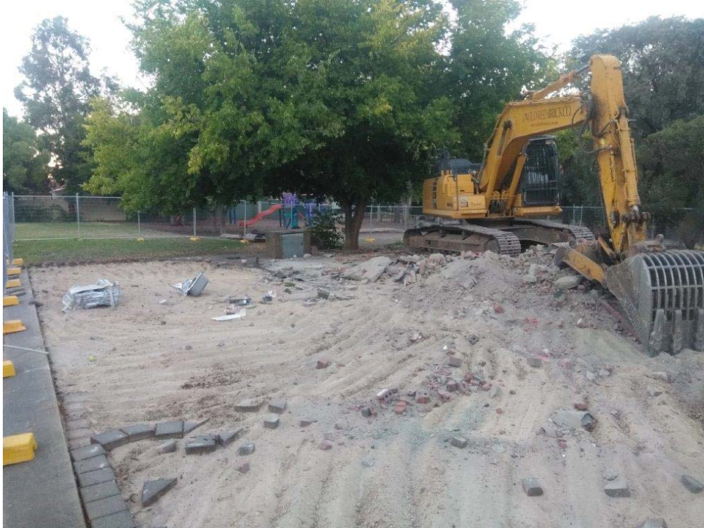
Figure 9, Demolition works tennis club house (4 March 2021)
