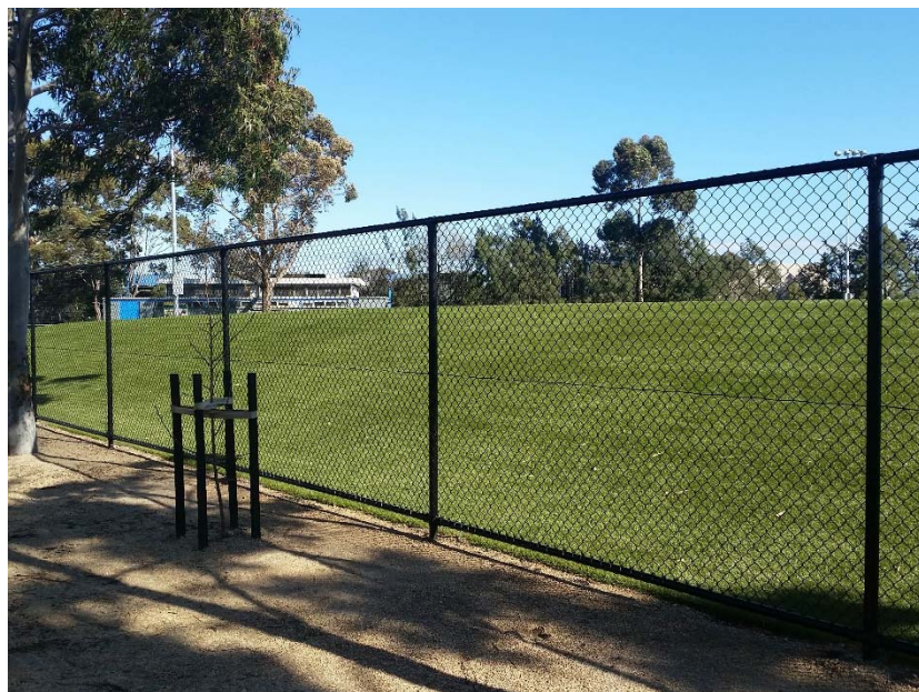
Figure 11, Chain link fencing
