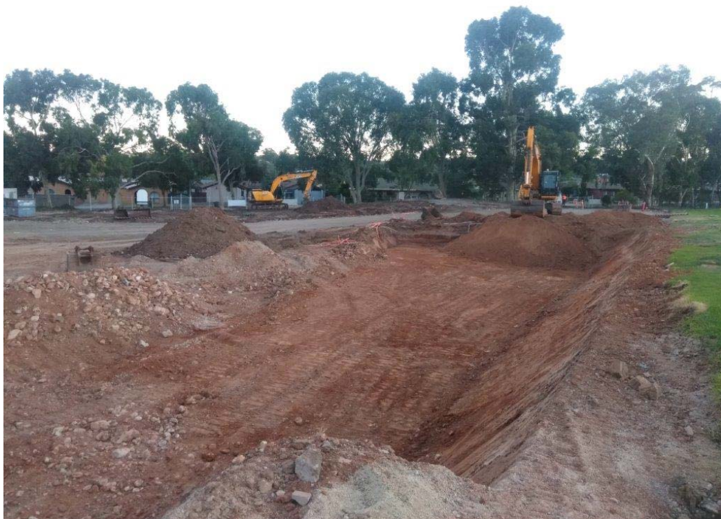
Figure 10, Preliminary civil works main building (4 March 2021)
