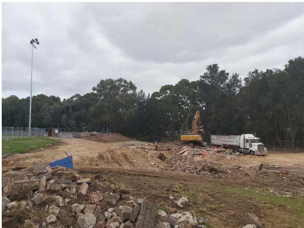
Figure 8, Demolition works main building (23 February 2021)
